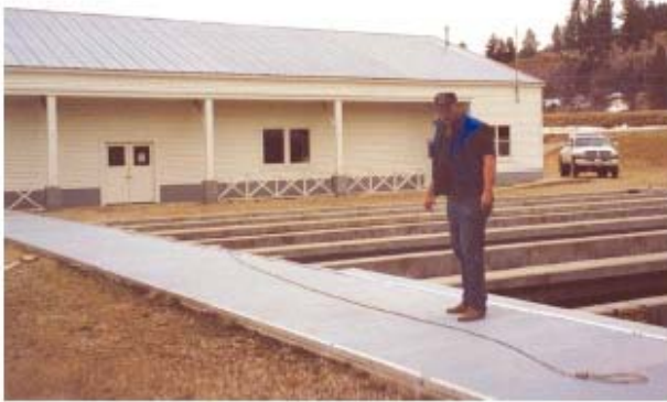
SAFPLANK® panels are used as tank covers at the Spring Creek Trout Hatchery in Lewistown, Montana. The lightweight panels allow easy access to the tanks and provide a safe walking surface for the staff.
