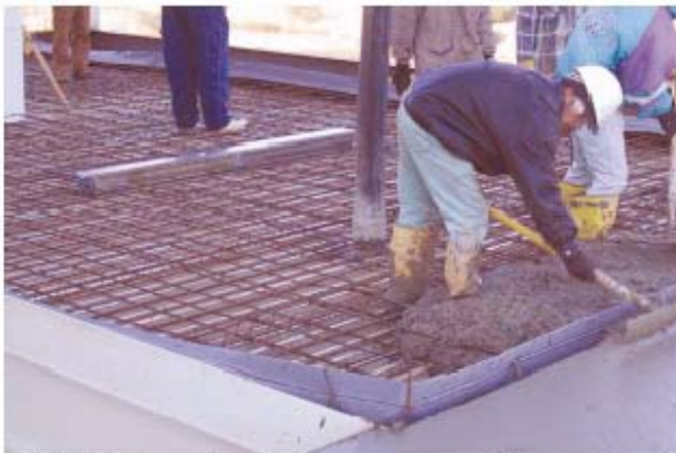
SAFPLANK®, when turned upside down, serves as an excellent concrete forming system in applications where corrosion and weight are construction concerns.
